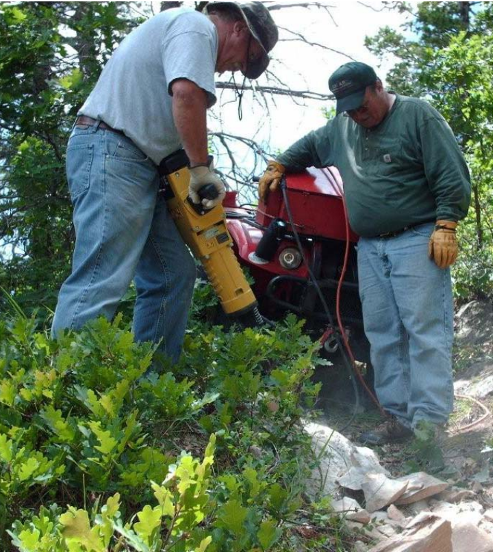
Mike Pehrson (l) and Brent Johansen bust up some rocks with our new electric rock hammer on the Gooseberry Trail.
